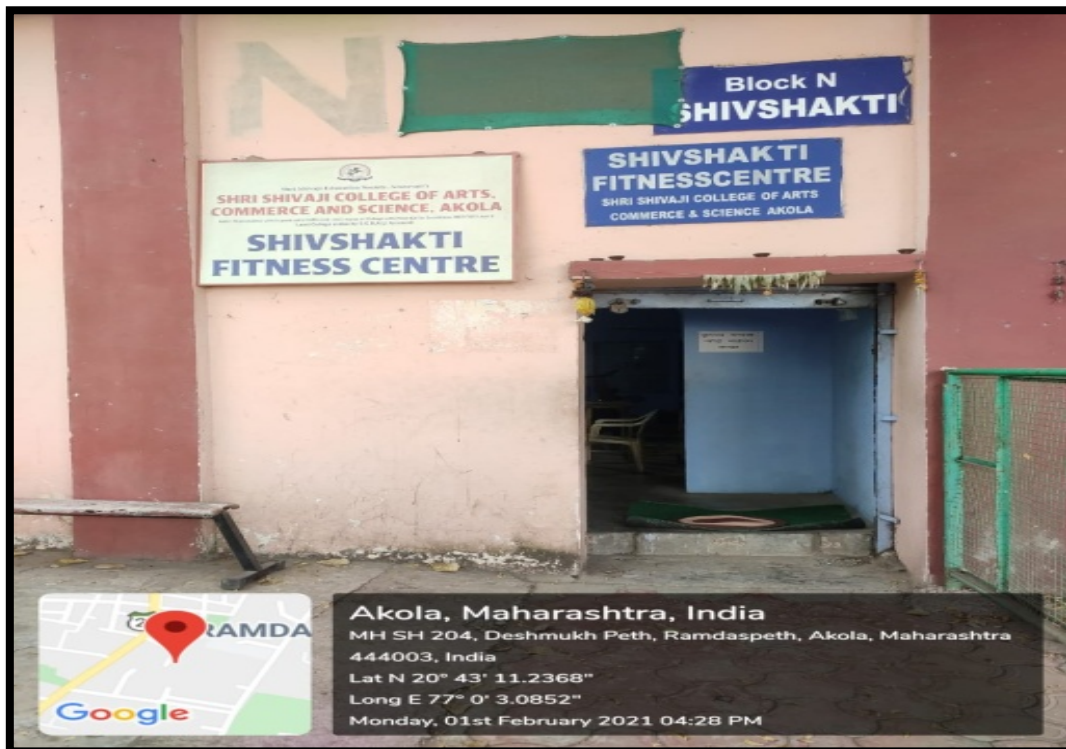
Front view of Gymnasium
